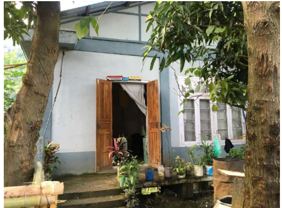
Pictures of completed In-situ unit at Zuangtui
