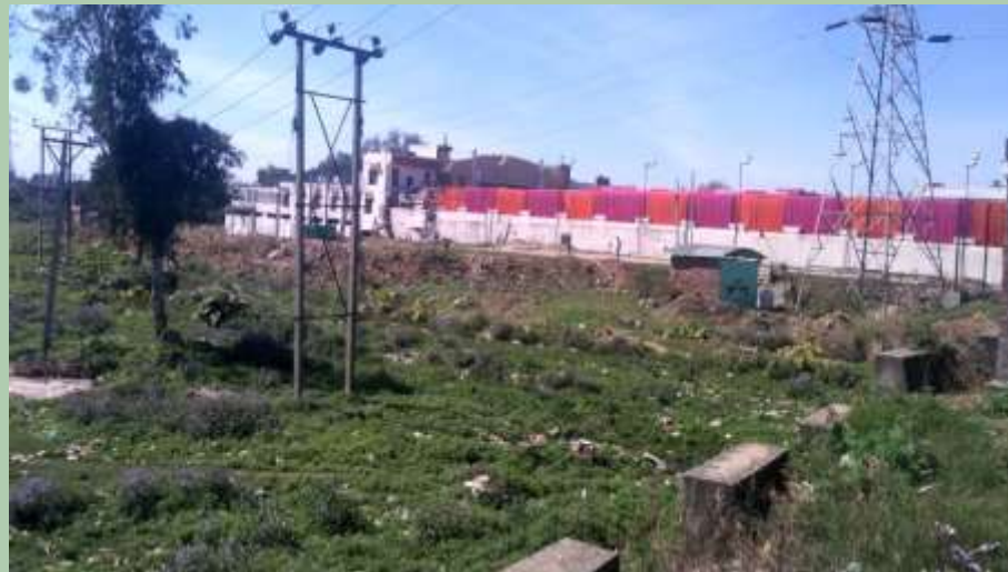
HT Lines over the site, kept open in layout
