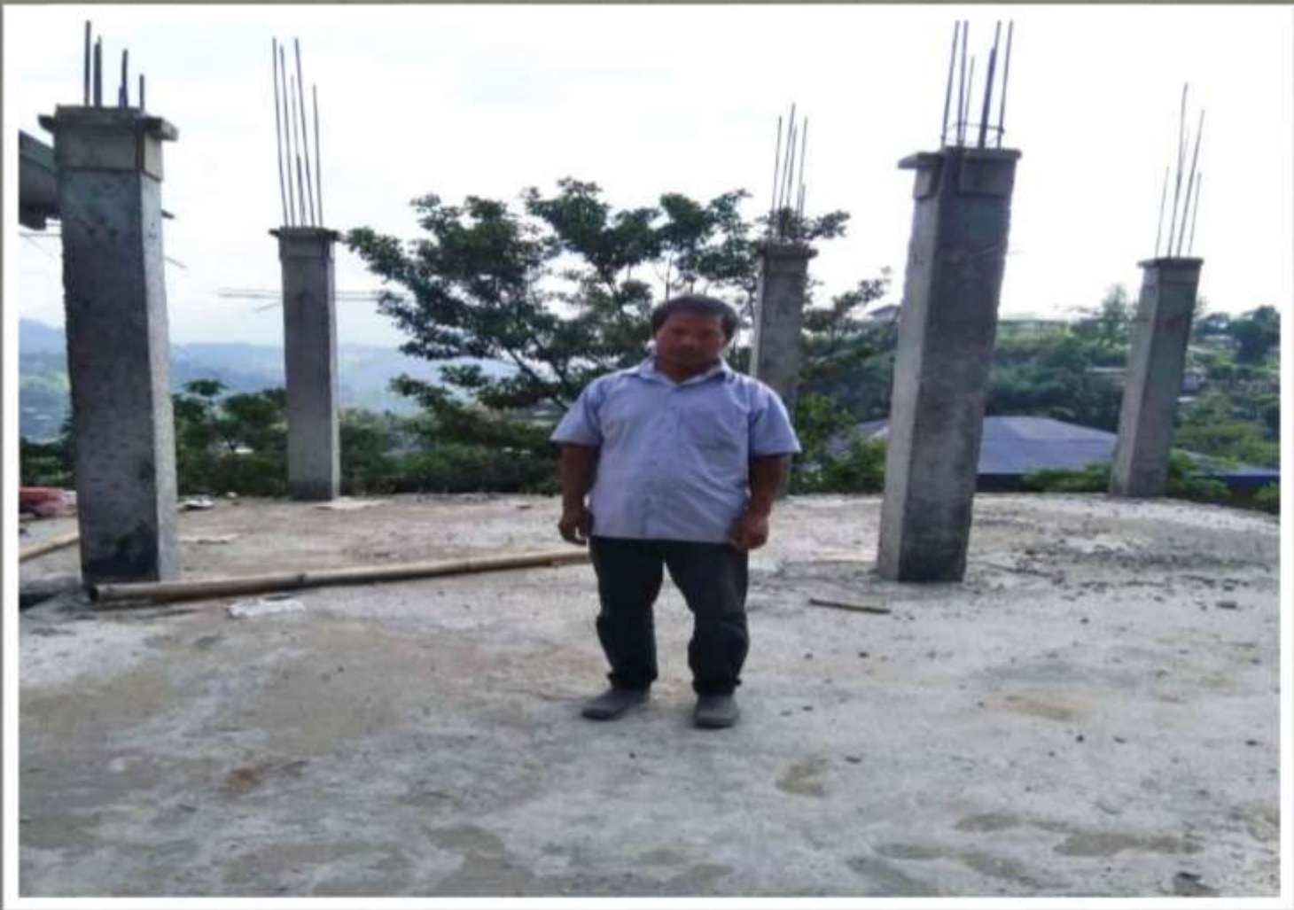
5) Name:- WARAN KHOMRANG Construction Stage:- Foundation Level
