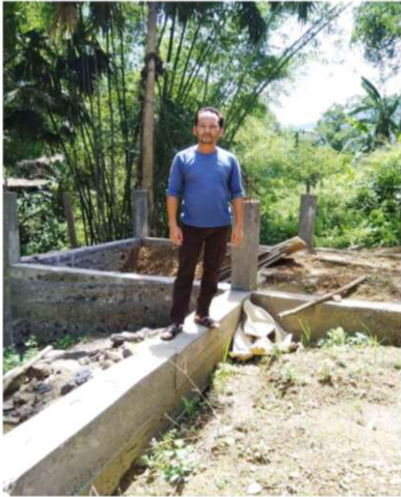
1) Name:- MAIKHUN MAMAI Construction Stage :- Foundation Level
