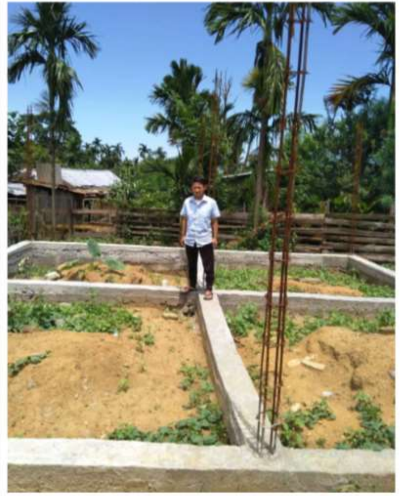
4) Name:- INGMAI SINGPHO Construction Stage :- Foundation Level
