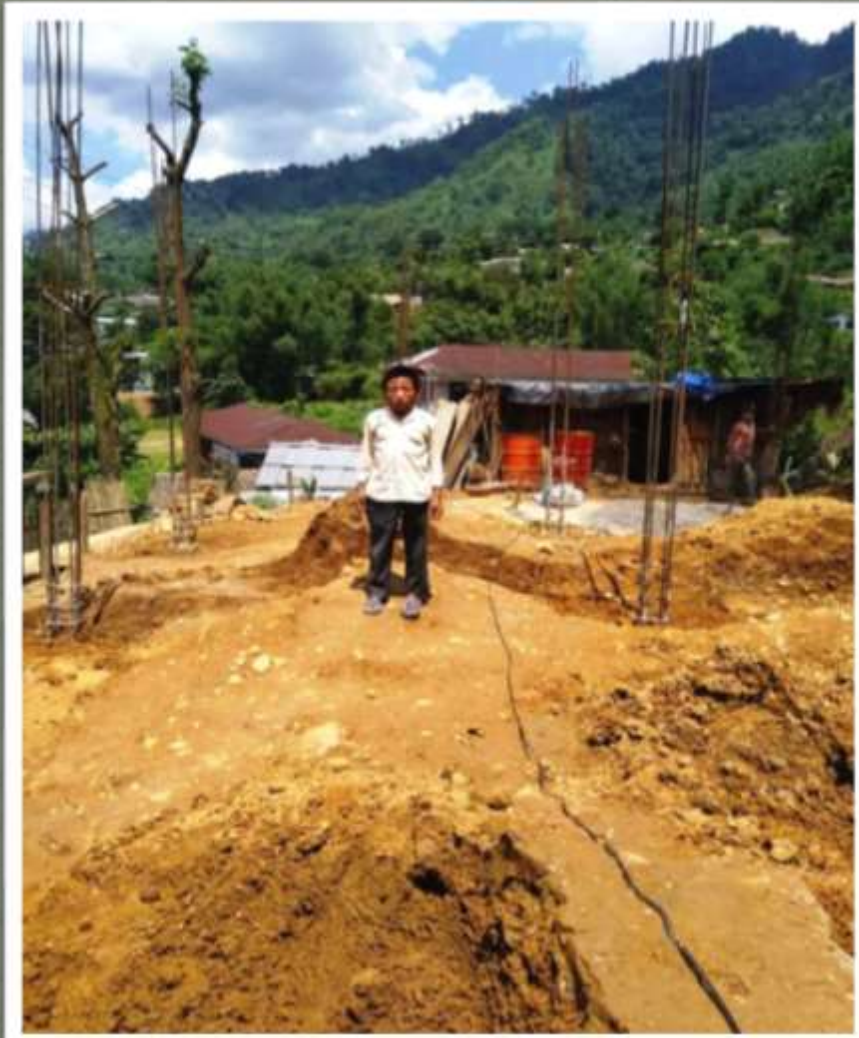
3) Name:- GOPANG NGEMU Construction Stage :- Foundation Level
