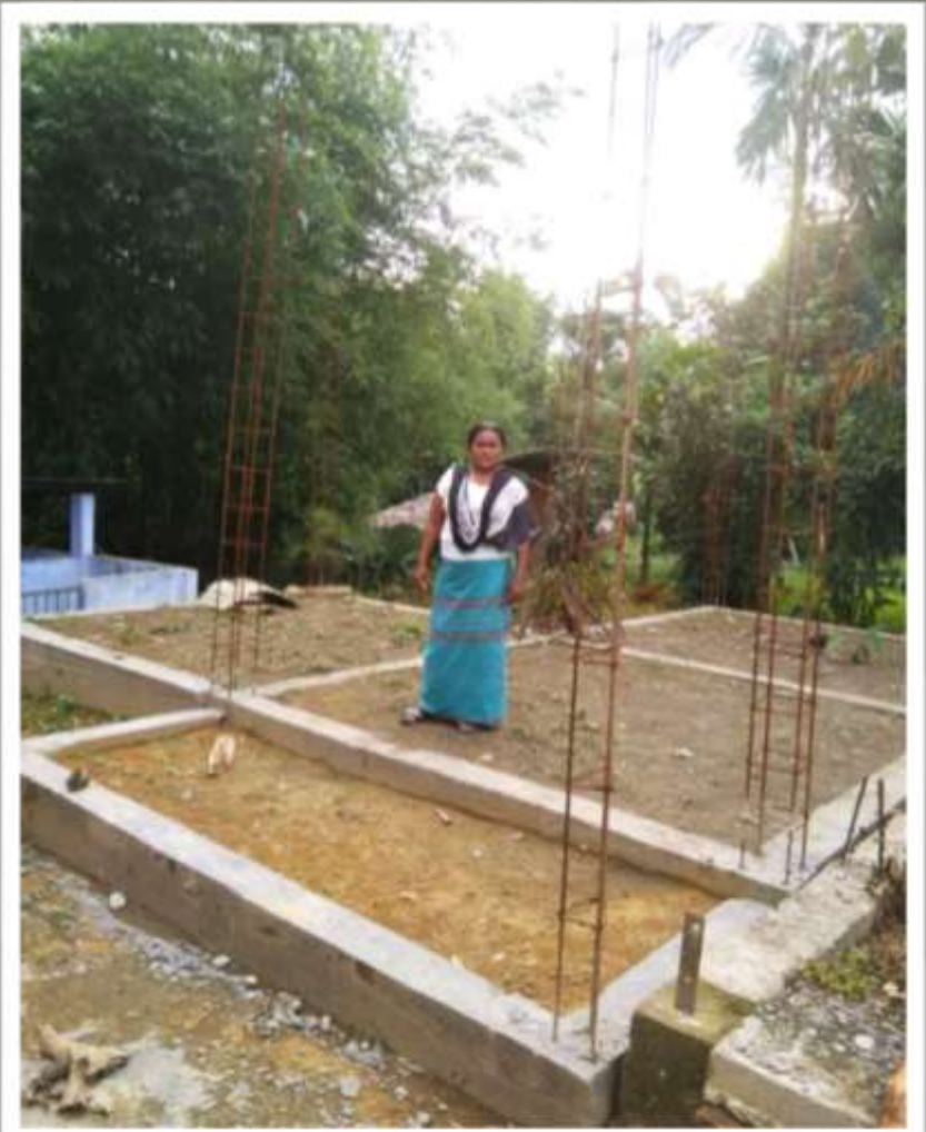
4) Name:- RUBON LONGRI Construction Stage :- Foundation Level
