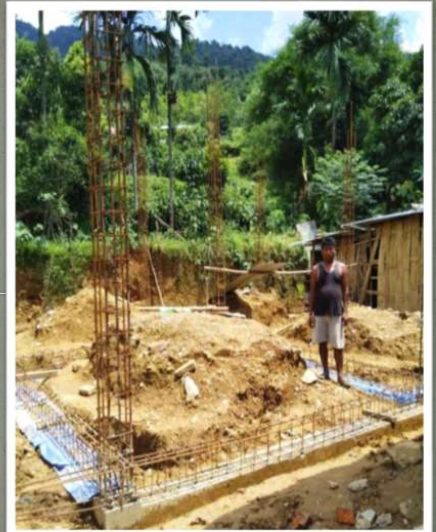
4) Name:- GANKAI NYEMDAM Construction Stage :- Foundation Level
