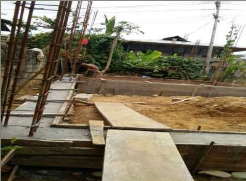
3). MEDDAK LONA, MEDICAL COMPLEX
