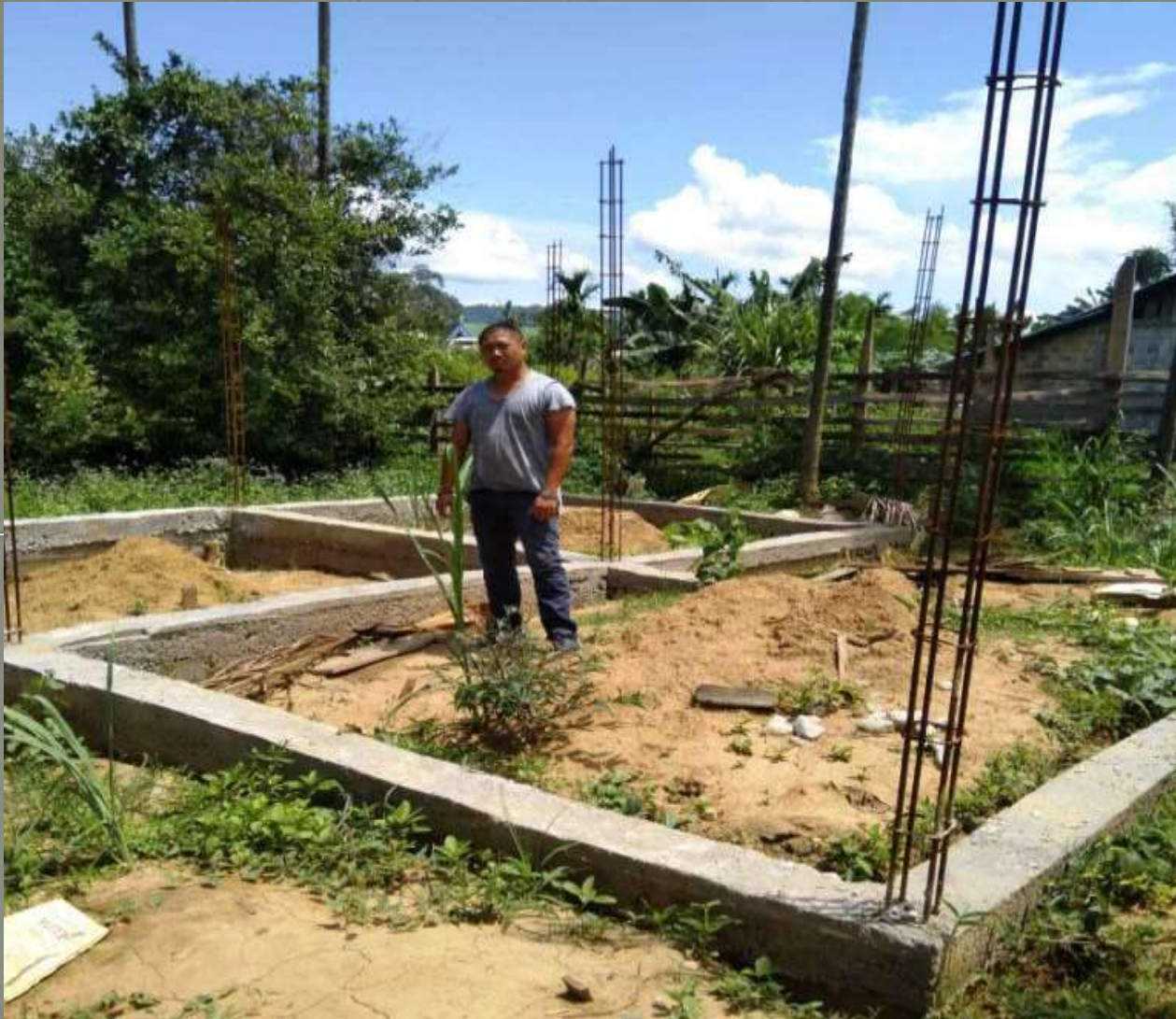
5) Name:- PARMESH LONGKHO Construction Stage :- Foundation Level
