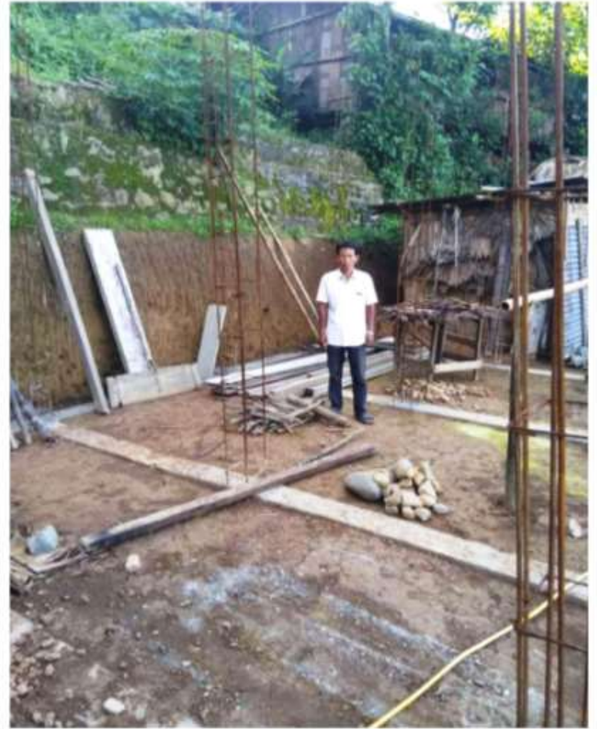
2) Name:- REDANG BO Construction Stage :- Foundation Level
