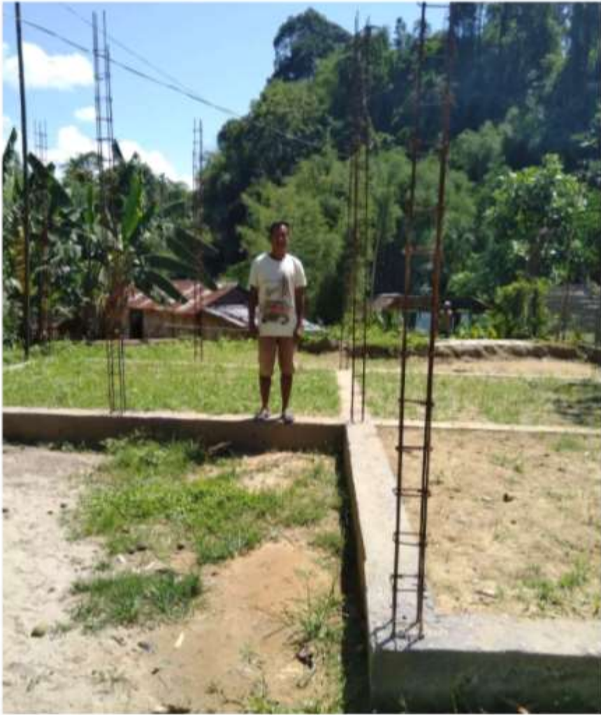
1) Name:- BUMCHA KIMSING Construction Stage :- Plinth Level
