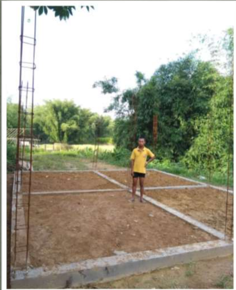
3) Name:- KHAMVANG LONGRI Construction Stage :- Foundation Level
