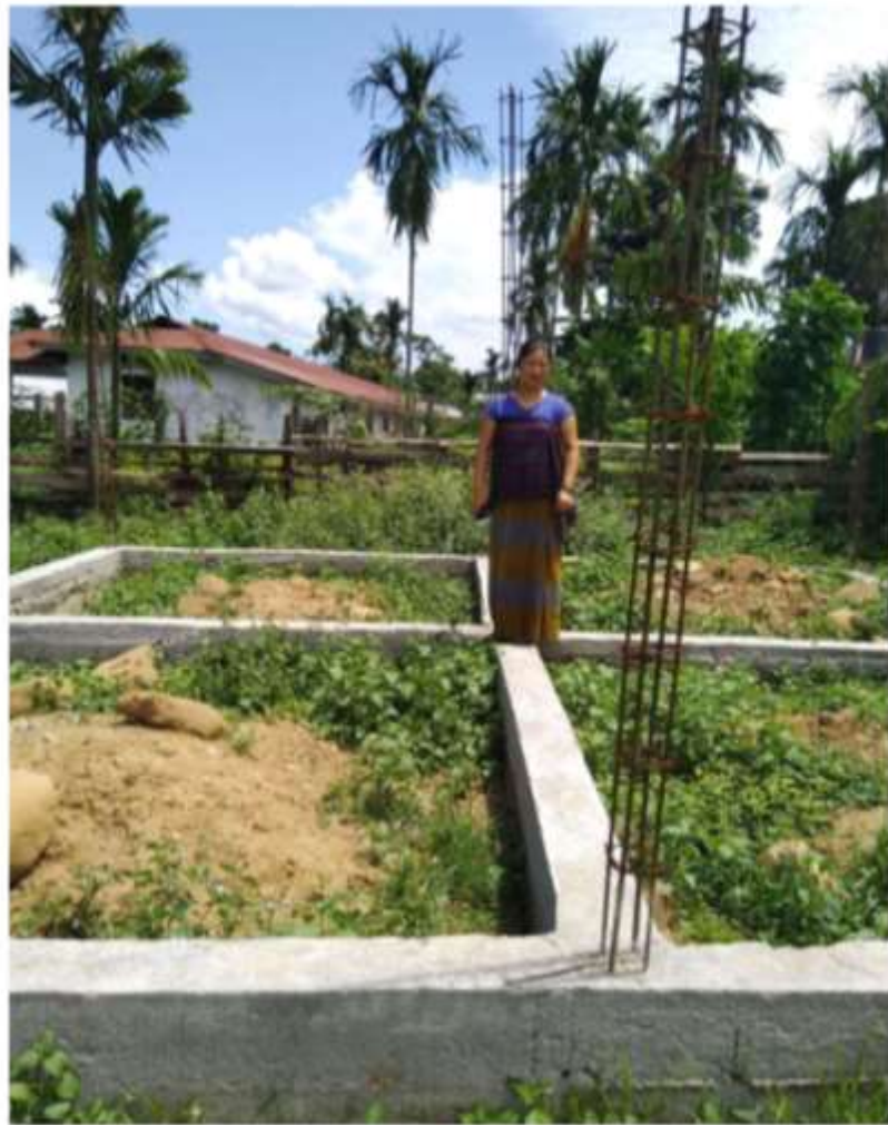
3) Name:- HUNTU MONI SINGPHO Construction Stage :- Foundation Level
