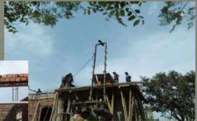
3. Roof level commenced
