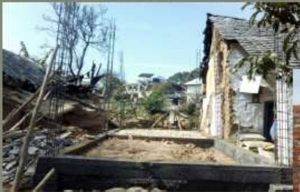
1. plinth level completed
