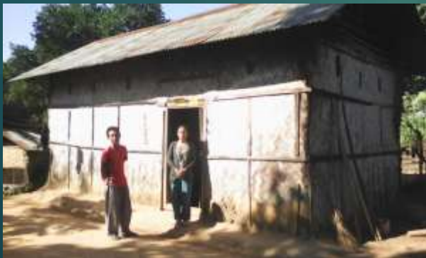
Beneficiary Name: Anile Ward Name: Veterinary Town: Jalukie BLC – New House Construction
