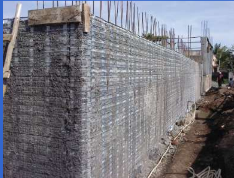
MONOLITHIC CONSTRUCTION WITH STRUCTURAL STAY IN PLACE STEEL FORM WORK SYSTEM
