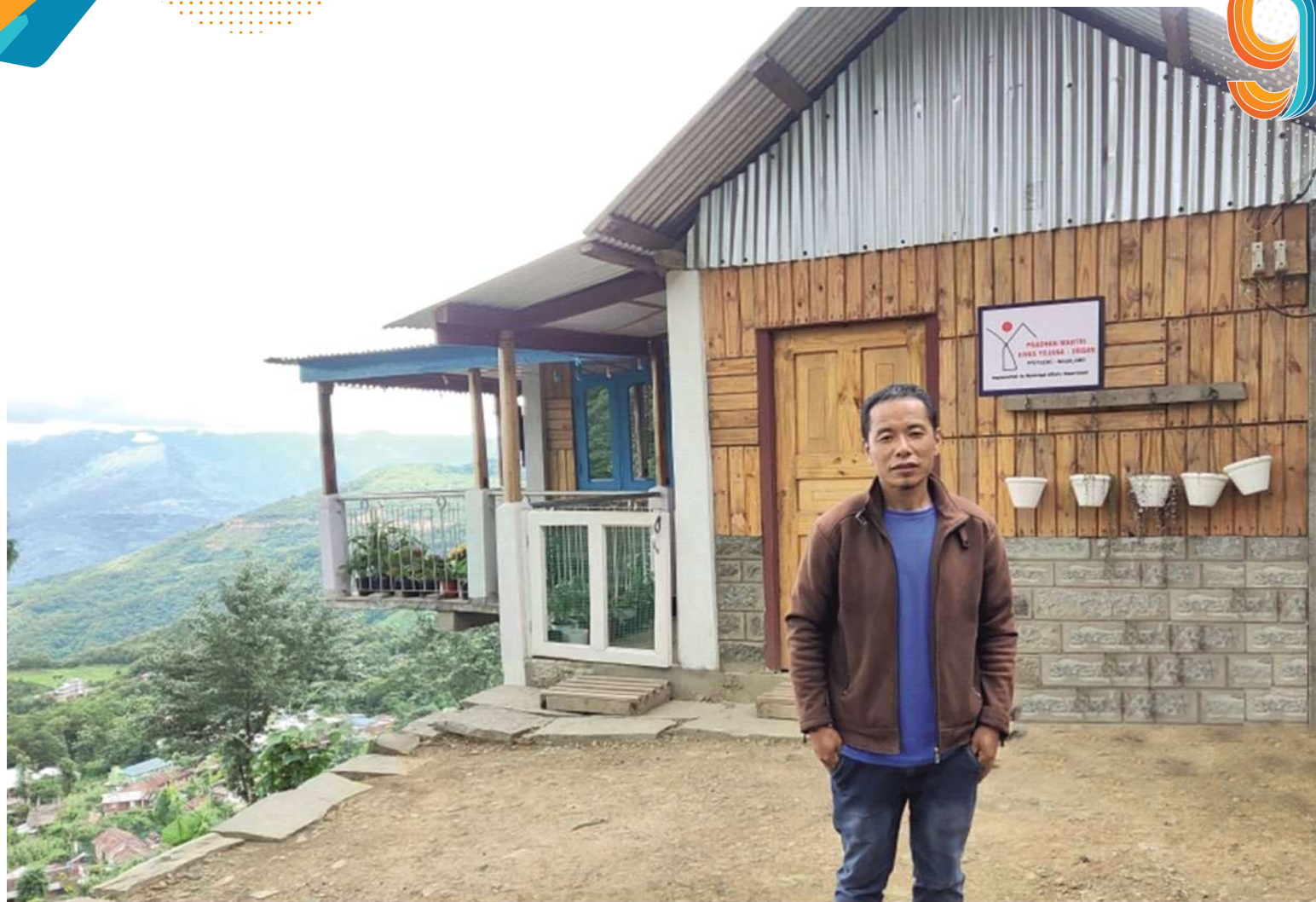
PMAY-U house of Keduwe Wetsah in Pfutsero, Nagaland
