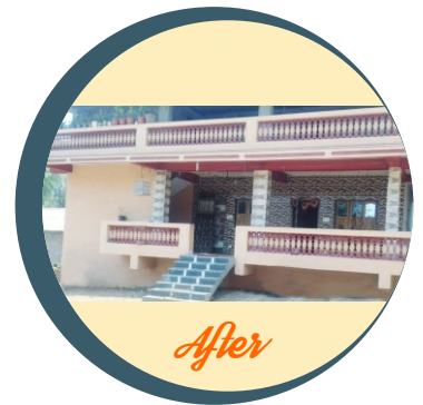
BLC House of Shri Pataliya, Silvasa, Dadra and Nagar Haveli
