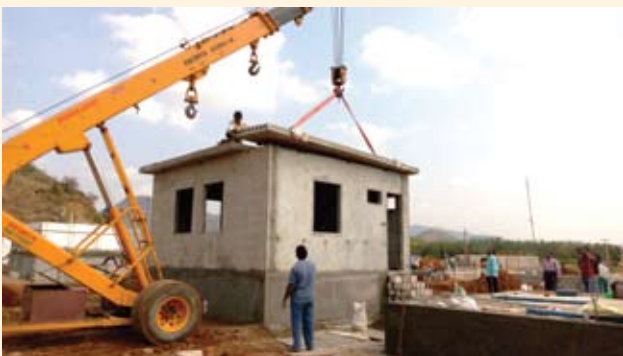
Houses being constructed using prefab technology by Govt. of Andhra Pradesh
